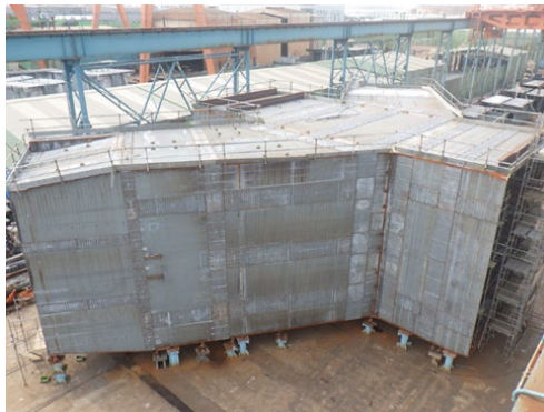
Fig. 8 Overall temporary assembly of the springing steel shell section (with the whole section overturned)
