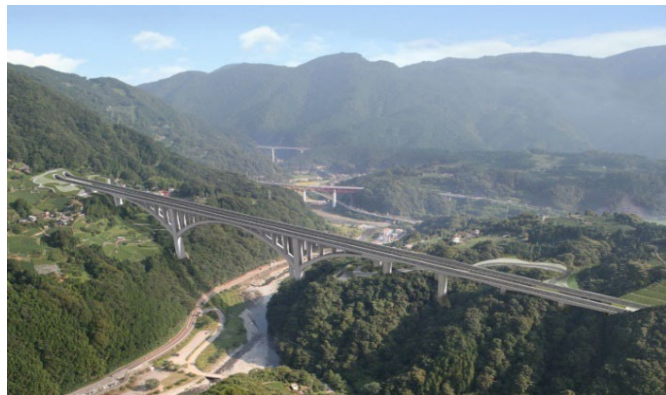
Fig.1 Rendering of the completed Kouchigawa bridge (Arch span length: 220m)
