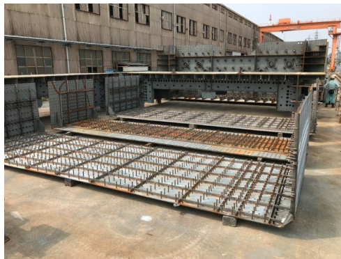
Fig. 11 Steel member blocks in pier steel formwork sections
