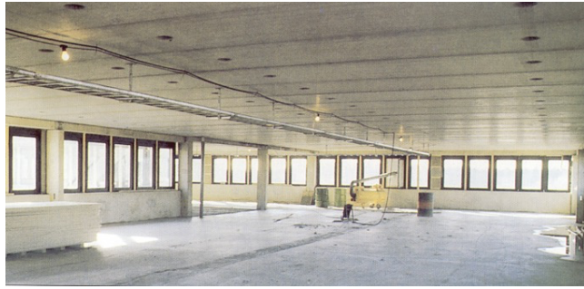
Figure 8. Hollow core floor for large open spaces [8]
