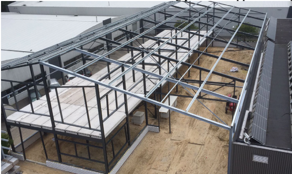
Figure 16. Precast mixed demountable structure. [7]
