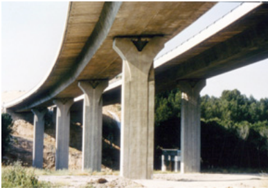
Figure 15. Continuous precast box beam bridge. [11]
