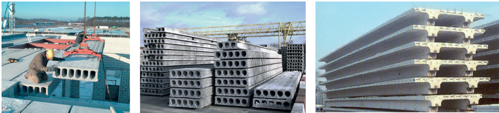
Figure 6. Precast hollow core and TT floors [8]
