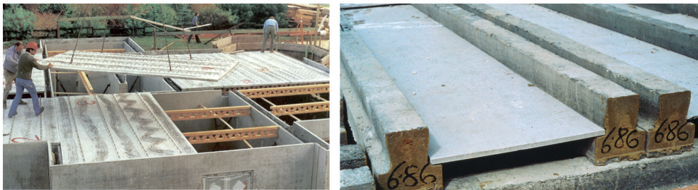
Figure 7. Precast composite floor-plate and beam and plate floors [8]
