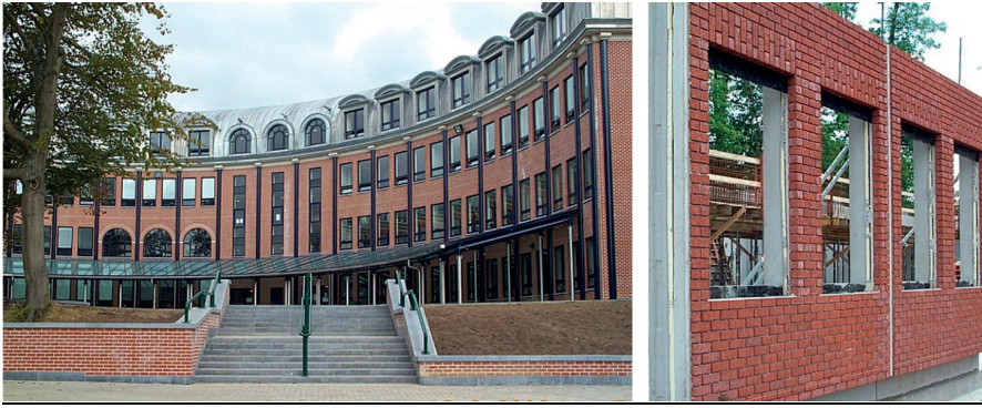
Figure 1. Precast panels with brick finishing. The European School, Uccle, Brussels [8]
