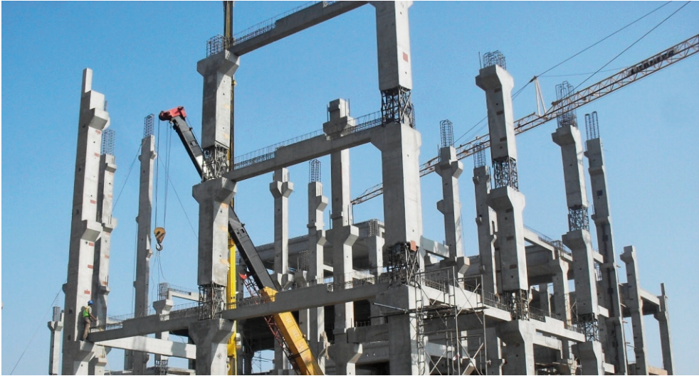
Figure 9. Precast building with monolithic connections for seismic areas. India. [16]
