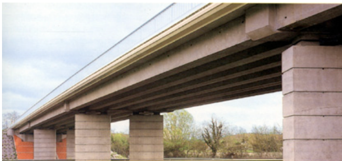
Figure 14. Continuous bridge with I beams. [11]
