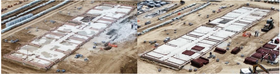
Figure 5 Slab-on-ground: (left) 1st concreting stage; (right) 2nd concreting stage
