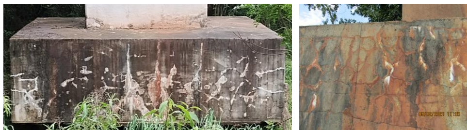
Fig. 2. Typical cracks identified on concrete pile cap of FA bridges
