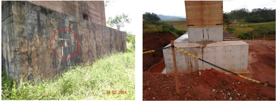
Fig. 5. Concrete pile caps of Soledade Viaduct, before and after intervention
