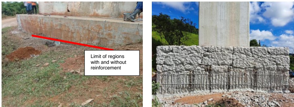
Fig. 6. Concrete pile caps of Viaduct 074-FA, during inspection and after cover removal
