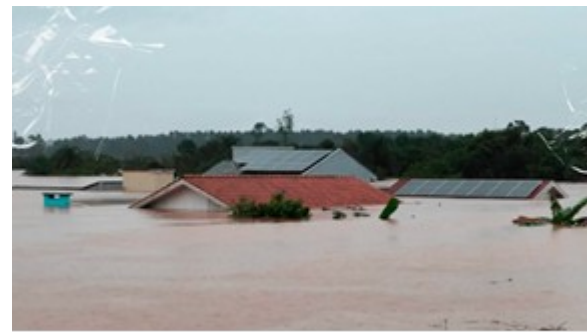
Figure 4. Properties flooded by flooding
