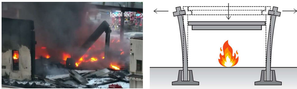
Fig. 4 Effect of thermal curvature on external columns (Fidenza fire – 2024) and sketch of loss-of-support mechanism for horizontal members
