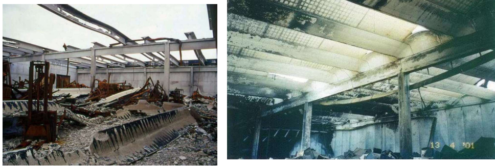
Fig. 2 Different performance of ribbed (left) and wing-shaped (right) precast elements in real fires
