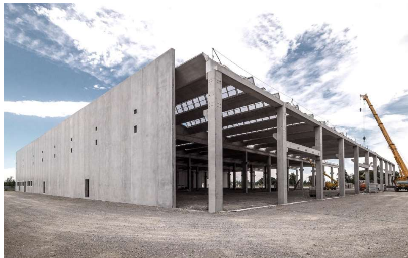
Fig. 1 Prototypal precast concrete industrial building
