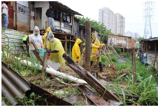
(a) Removal of old unit
