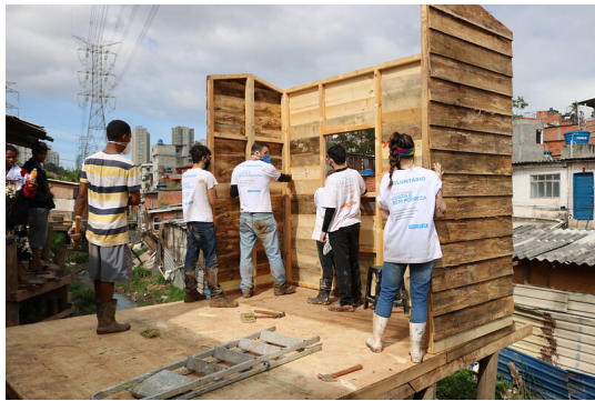
(c) Construction of new unit
