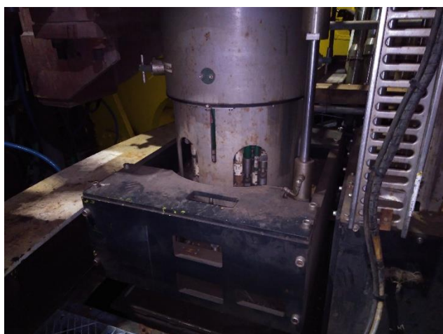
Figure 8. Example of a confined industrial environment
