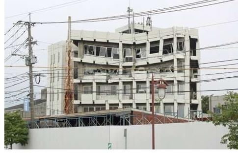
Fig. 2 City Hall Main Building with intermediate-story collapse [3]
