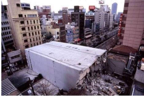
Fig. 1 Building that collapsed sideways and blocked the road [2]
